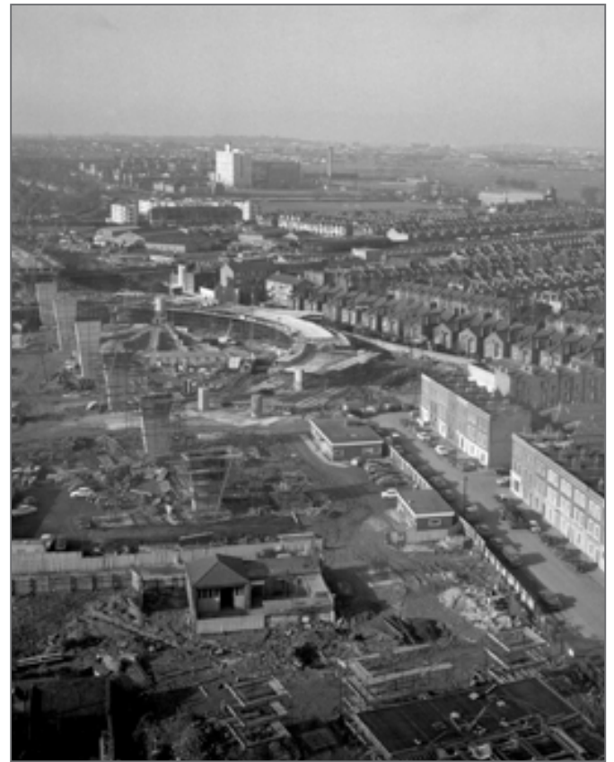
The A40 (M) Westway, a 2.5 mile elevated dual carriageway in West London running from Paddington to North Kensington under construction during the period 1964-1970. It was built to relive congestion at Shepherd's Bush caused by traffic from Western Avenue.
