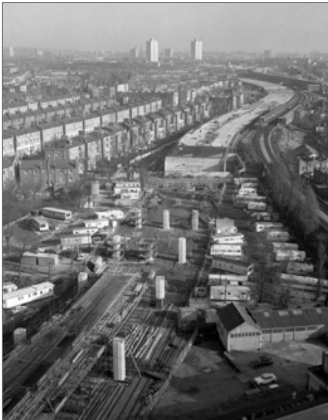
The A40 (M) Westway, a 2.5 mile elevated dual carriageway in West London running from Paddington to North Kensington under construction during the period 1964-1970. It was built to relive congestion at Shepherd's Bush caused by traffic from Western Avenue.
