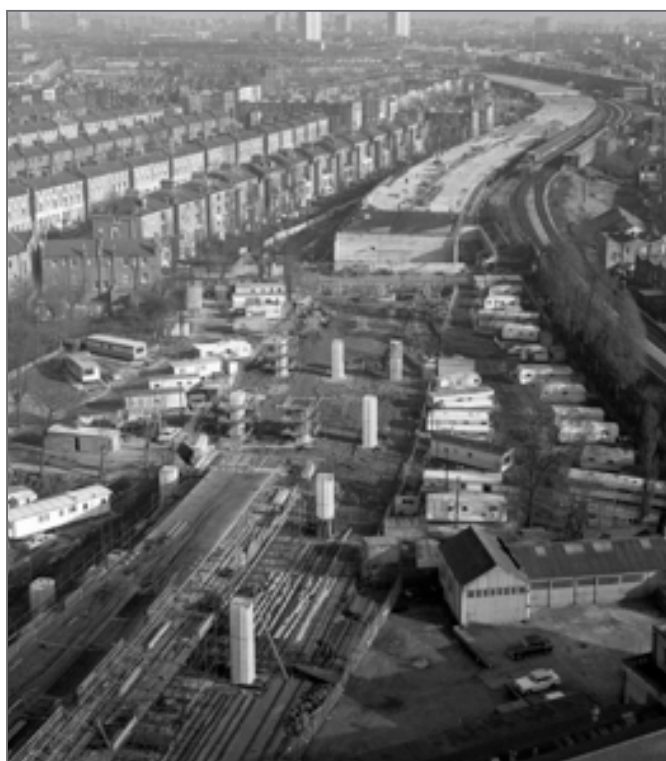
The A40 (M) Westway, a 2.5 mile elevated dual carriageway in West London running from Paddington to North Kensington under construction during the period 1964-1970. It was built to relieve congestion at Shepherd's Bush caused by traffic from Western Avenue.
