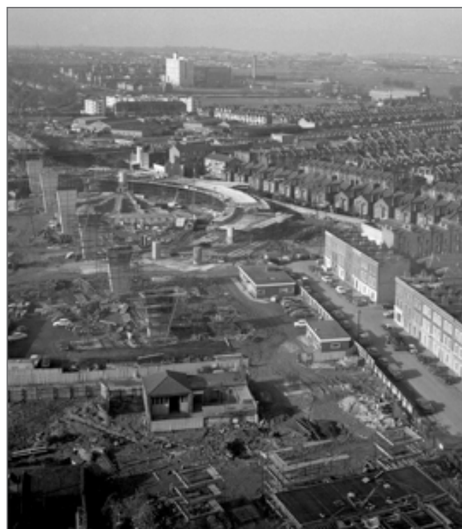
The A40 (M) Westway, a 2.5 mile elevated dual carriageway in West London running from Paddington to North Kensington under construction during the period 1964-1970. It was built to relieve congestion at Shepherd's Bush caused by traffic from Western Avenue.
